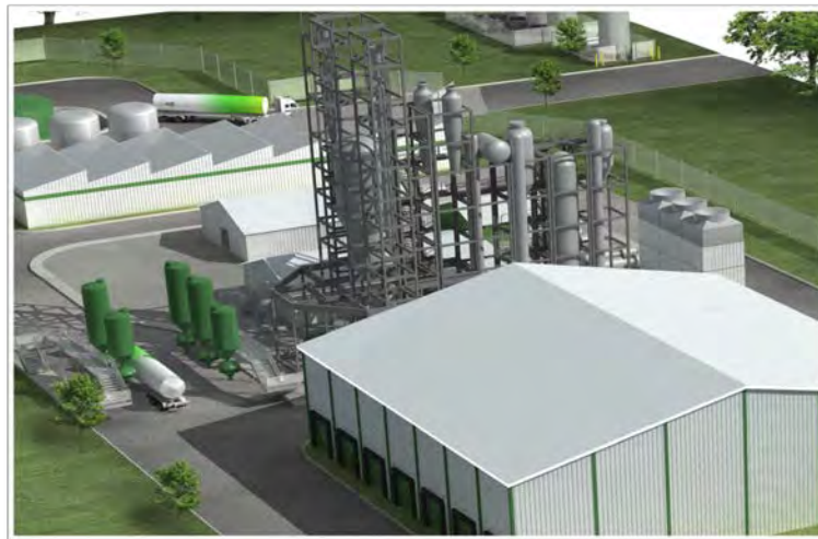
Enerkem Pontotoc, Mississippi 300 TPD MSW Gasification to Ethanol Project (Expandable to 600TPD) 10 Million Gallons Ethanol/Year Construction Start 2013; Operation 2014/2015
