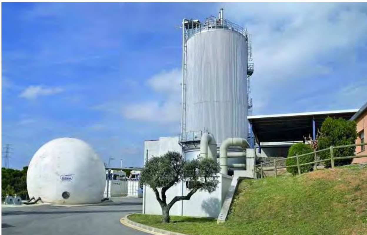
DRANCO Facility Terrassa, Spain 25,000 TPY Biowaste; Electricity December 2006
