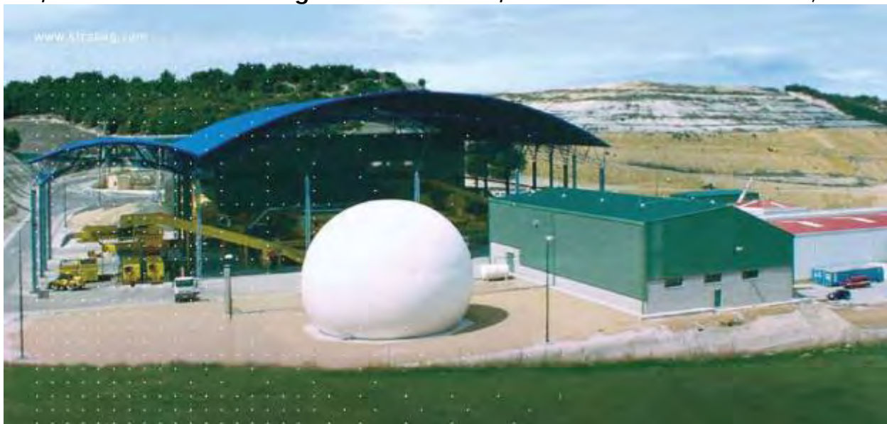
STRABAG Facility Valladolid, Spain
