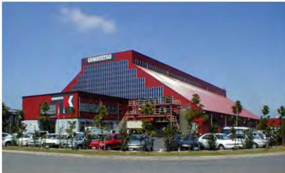
IWT Thermoselect Gasification – Chiba, Japan 330 TPD Operating since 1999
