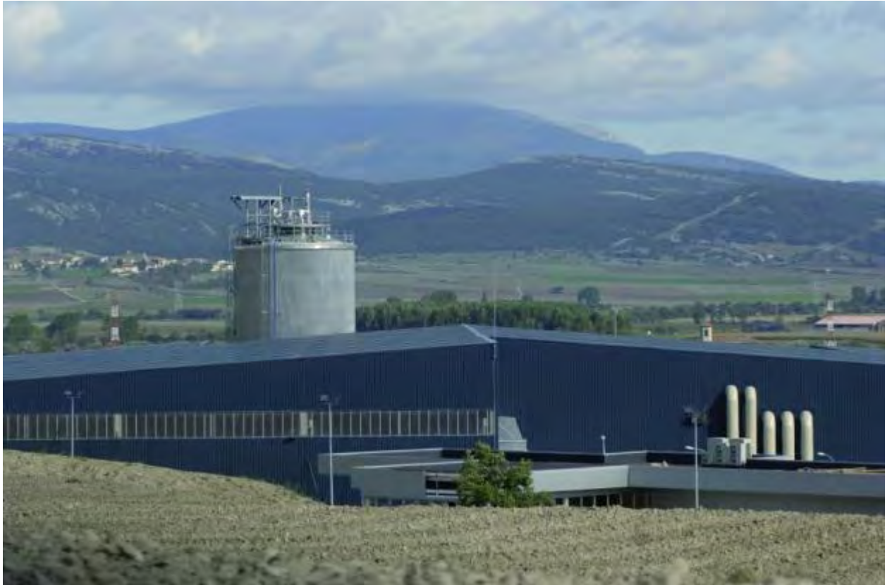
DRANCO Facility Vitoria, Spain 330 TPD Mixed MSW 2006
