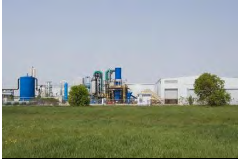
Plasco Trail Road Plasma Gasification to Electricity Facility, Ottawa, Canada 150 TPD MSW, Demonstration Facility Operating since 2007, Recently Permitted/Upgraded for Commercial Use in 2011/2012, 4MW Electric Generating Capacity
