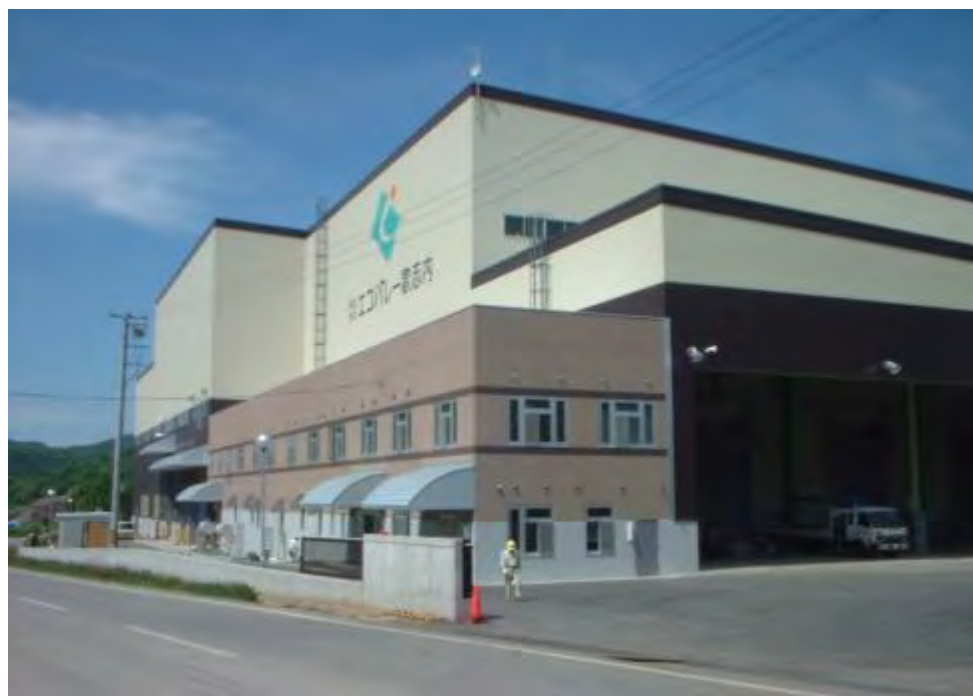
Westinghouse Plasma Gasification System, Utashinai, Japan 300TPD Mixed MSW (or 165TPD Auto Shredder Residue), Electricity Commercial Operation in 2003
