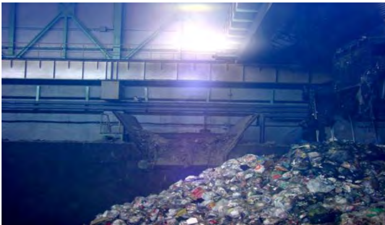
Waste in Pit, JFE/Thermoselect Gasification Facility, Kurashiki, Japan, 610 TPD Mixed MSW, Commercial Operation since 2005
