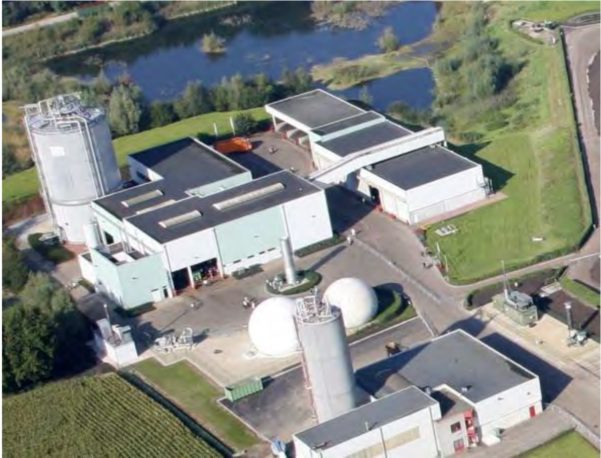
DRANCO Facility Brecht, Belgium 20,000 TPY Biowaste (Brecht I) 50,000 TPY Biowaste (Brecht II) Electricity July 1992 (Brecht I) January 2000 (Brecht II)
