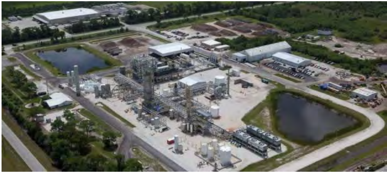
INEOS BIO INDIAN RIVER, FLORIDA, GASIFICATION TO ETHANOL FACILITY OPERATING SINCE FALL OF 2012 ON GREEN WASTE, ETHANOL PRODUCTION 1 ST QTR 2013 PREPROCESSED MSW TESTING IN FIRST HALF OF 2014 (300 TPD DRY FEEDSTOCK, 8 MILLION GAL/YR ETHANOL, 6MW GROSS POWER)
